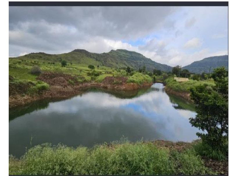
Earthen Nala Bunds strategically slow surface runoff to retain water
