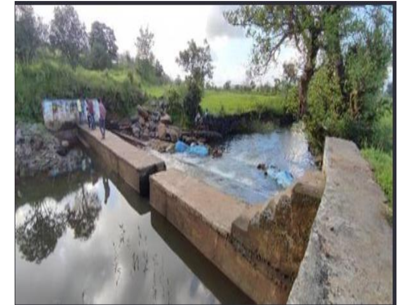
Checkdams slow water flow and increase soil moisture retention
