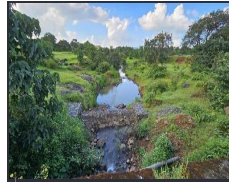
Core-wall Gabions stabilize soil and trap sediment along contours
