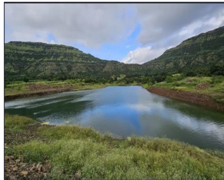
Percolation Tanks collect runoff, promoting groundwater recharge
